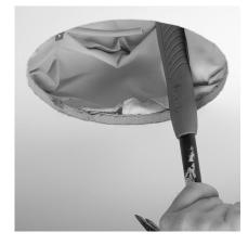
Using an inverted hammer handle (or similar blunt object), push it up in to the firehood & move it around to completely open out the cover.
